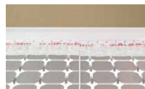
4. Laying of R883-1 insulation panel with coupled aluminum heat transfer profile
