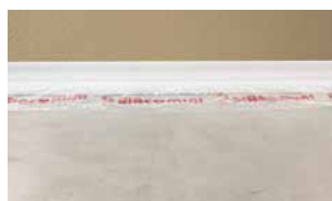
1. Laying of wall edging strip
