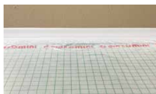
2. Laying of steam barrier polyethylene sheet
