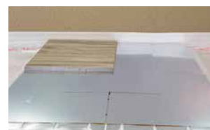
8. Laying of surface finish (floating on special mat recommended)
